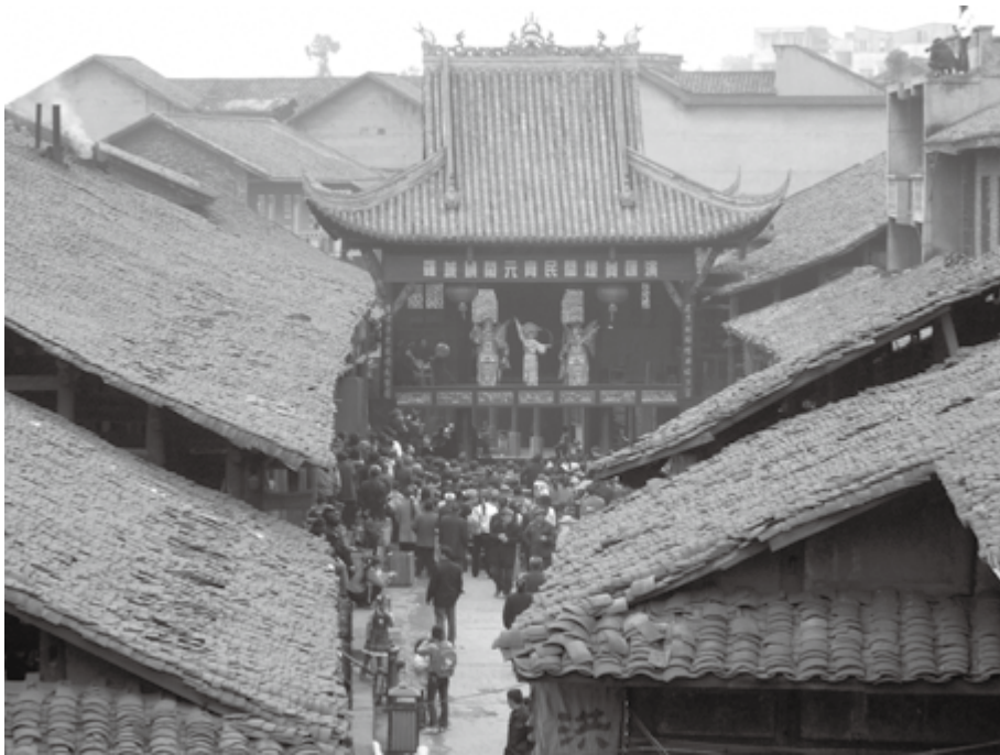
■ Ancient Xi Tai of Overpass Tower in Luocheng Town, Jianwei County, Sichuan. Photographed by Du Jianhua
